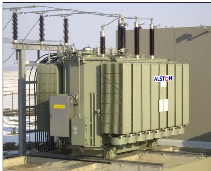
**Fig. 5:** Hermetically sealed power transformer 80 MVA / 110 kV
