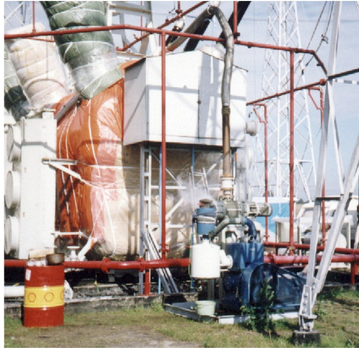
Fig. 2. View of the on – site drying stand. On the first plane – vacuum pump set
