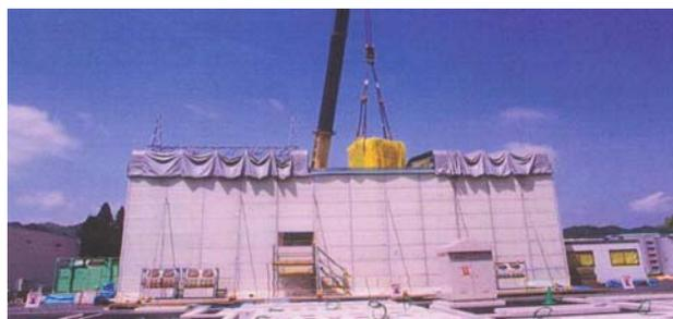
Fig. 10 Coils being reassembled in dustproof, low-humidity house
