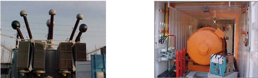
Figure 3 – Transformer (400MVA, 500kV) under HV On-site Testing and Motor-Generator Group (2MVA)
